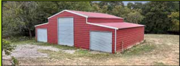
HOUSE & LARGE BARN/SHOP on 15 ACRES (M/L) NEAR LAKE TEXOMA - $549,000
