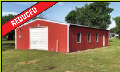
COMMERCIAL BLDG ON 4 LOTS in KINGSTON - $139,000
